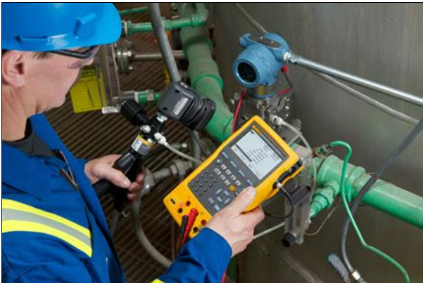
Fig 5: Manual calibration work in progress.
