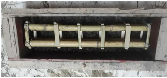
Fig 8: Casting of Bamboo Reinforced Concrete beam (200 × 200 × 800) mm
