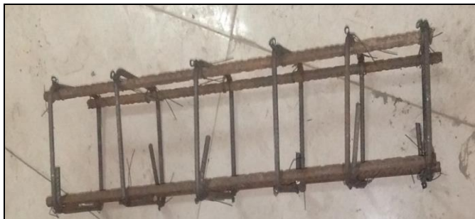
Fig 4: Bar bending of Steel for Reinforcement
