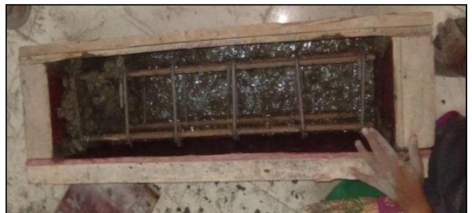
Fig 7: Casting of Steel Reinforced Concrete Beam (200x200x800) mm
