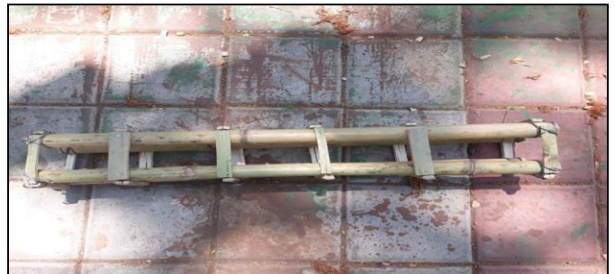
Fig 6: Bar bending of Bamboo for Reinforcement
