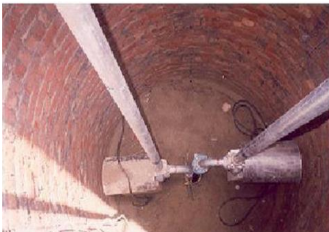
Fig 2: A typical cut-down pump
